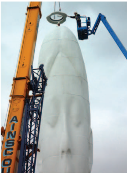
Figure 6: Positioning of final precast unit.
